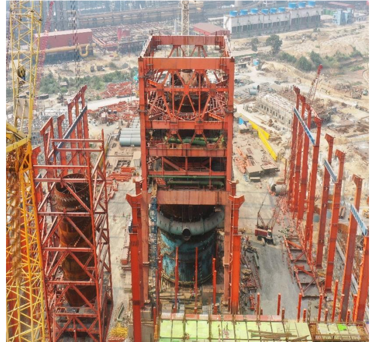
Blast Furnace under construction
