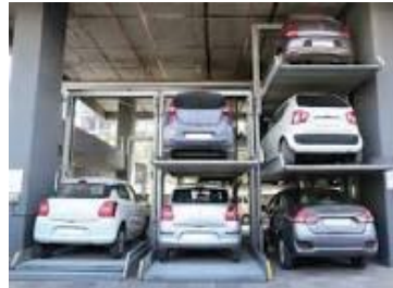
Parking Structural Support
