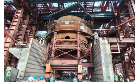
Converter vessel erected at SMS
