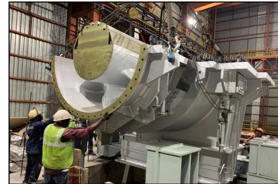
Top Recovery Turbine erection at BF
