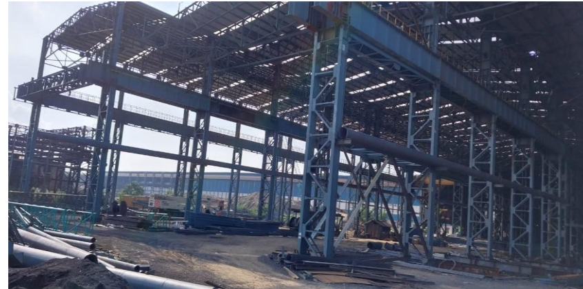
SMS-2 construction at BPSL
