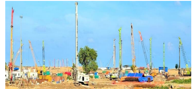
Piling in progress for Pellet Plant in Odisha
