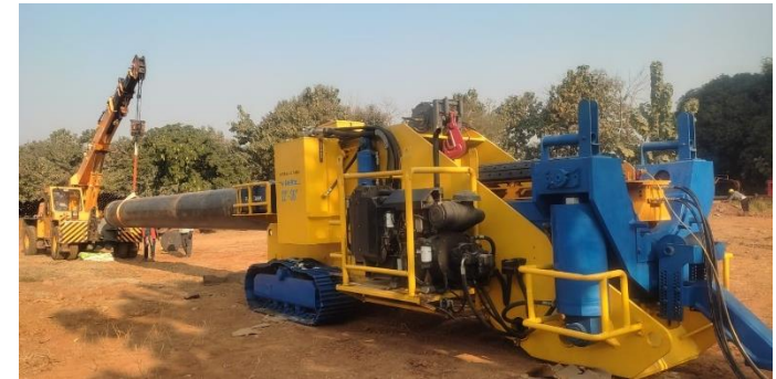
Slurry Pipeline: Bending Pre-Qualification Trial
