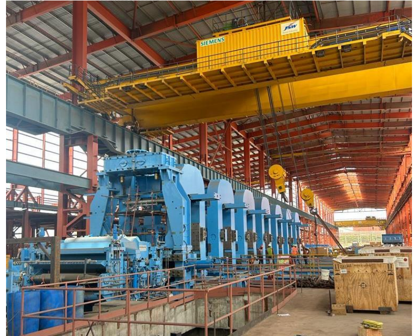
HSM under construction at Vijayanagar
