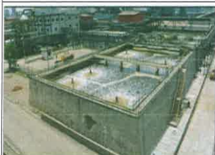
MBR+RO+ZLD plant at Coke Oven (4000 m3/d)
