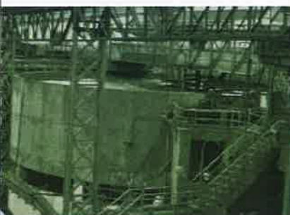
CO2 injection system at SMS
