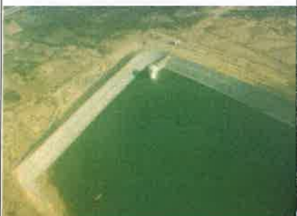
Raw water reservoir (35 Mn m3)
