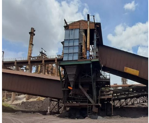
Source Mounted Dedusting at Sinter Plant
